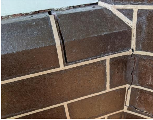
Close-up of low brickwork wall to the entry verandah showing significant cracking.
