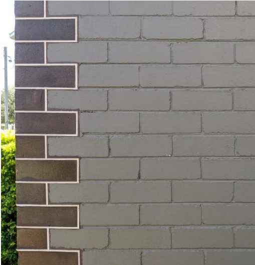
Close-up of brick wall to south elevation showing the change in brick types. The brick to the left is part of the recent renovations to brick to the right is original.
