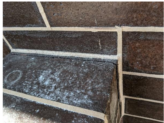
Close-up of low brickwork wall to the entry verandah showing significant cracking.
